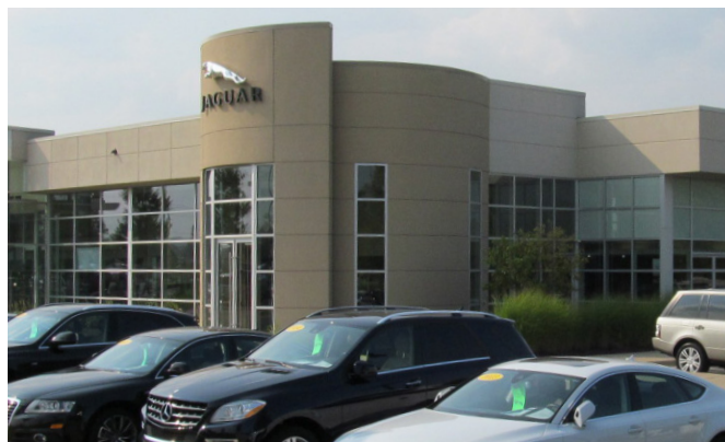
Figure 5: 9-year field test at Jaguar Land Rover building in Macomb, Michigan.
