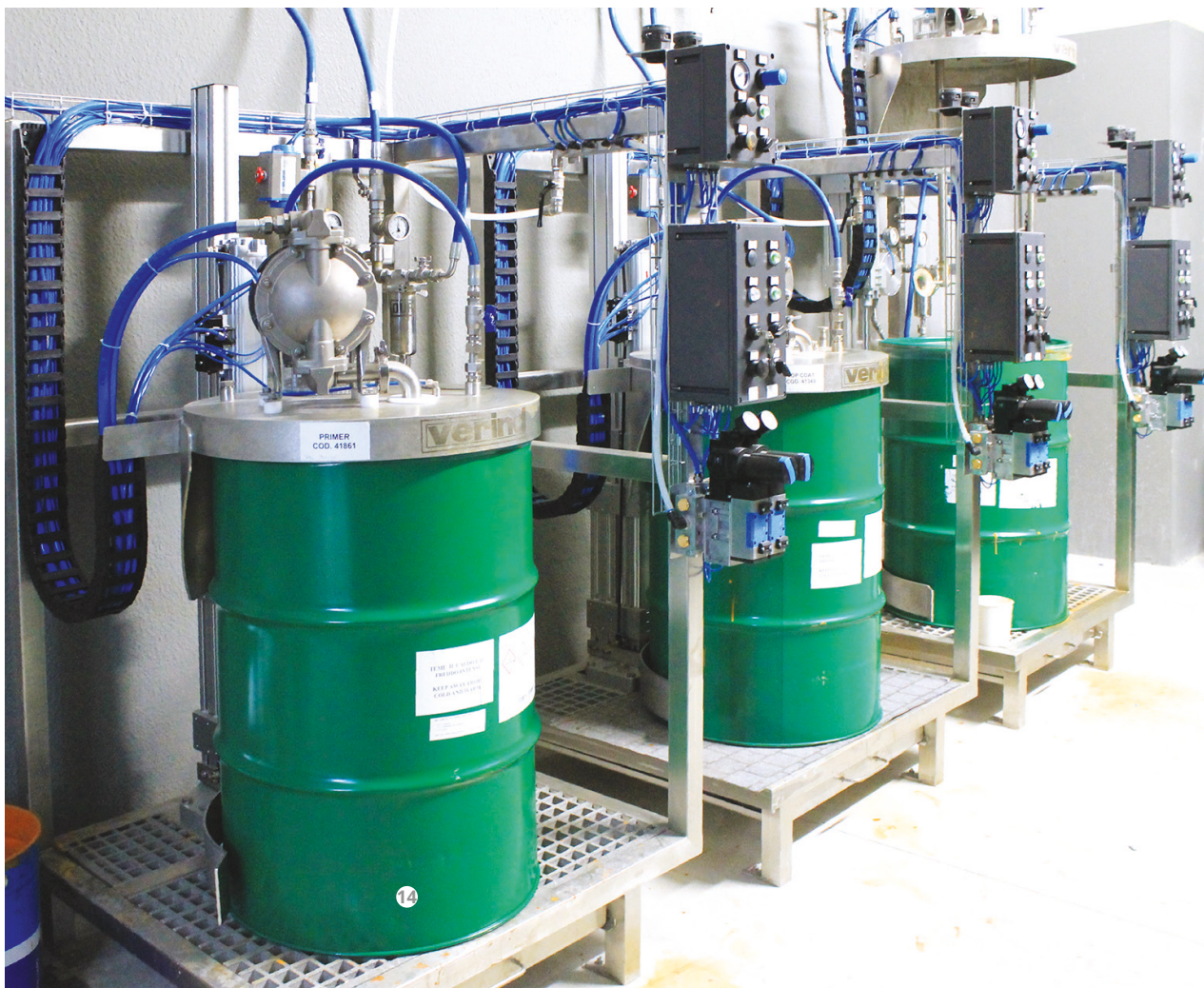
Figure 14: The pumping and recirculation unit of the coating products created by Verind/Dürr.
