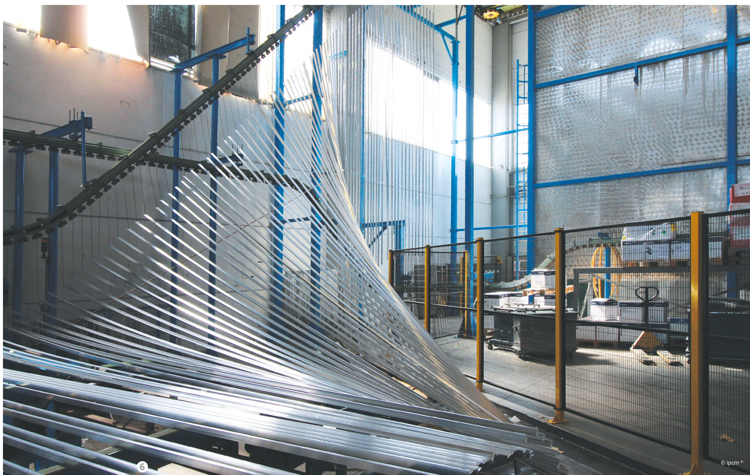
Figure 6: The profile loading area and the entrance to the 10-stage pre-treatment tunnel.
