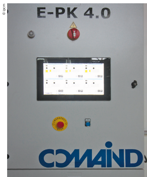
Figure 10: Mascar installed a control panel to manage the system and detect anomalies.
