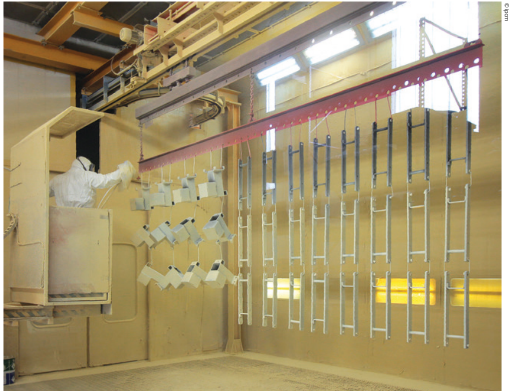
Figure 3: Manual primer application.
