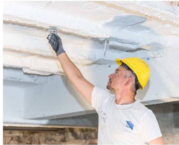
Measurement of the wet film layer thickness directly after the application.
