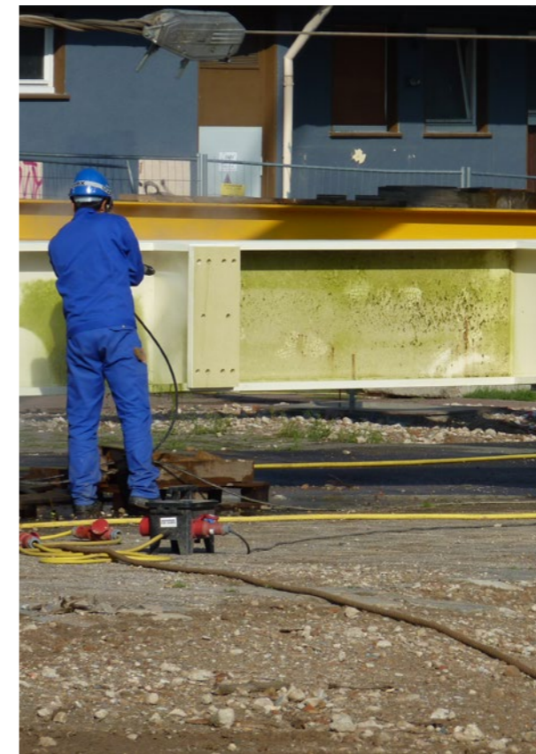
High-pressure cleaning of the steel beams
