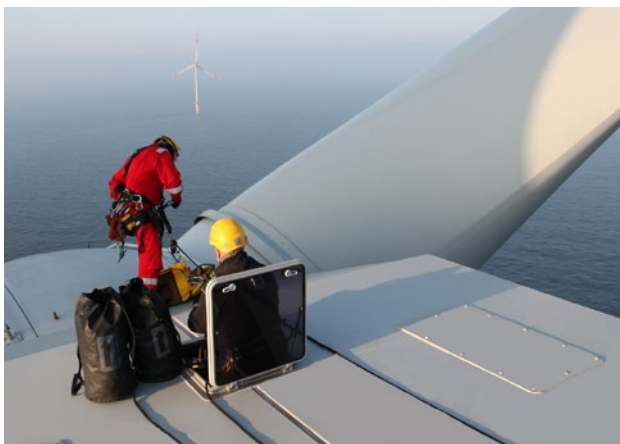
Figure 7: Wind blade inspection
