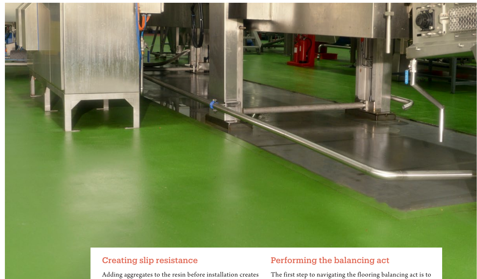
Right FasTop installed at a food production plant. © Steve Parkin
