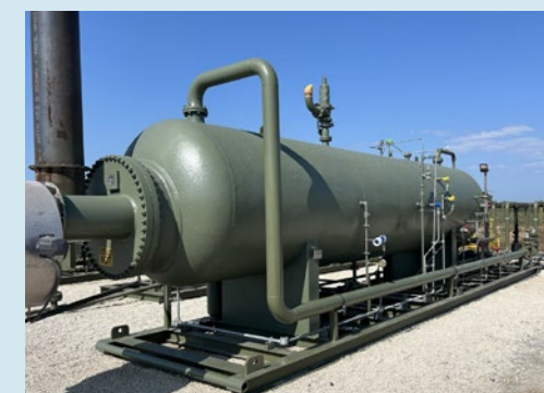
Figure 2 Like storage tanks, heater treaters can be covered with TICs in place of traditional insulation systems to maintain process heat. This unit was first primed with Heat-Flex ACE for corrosion protection (top) and then covered with the TIC Heat-Flex AEB (middle) to lock in process heat before being top coated (bottom) for aesthetic and durability purposes.
