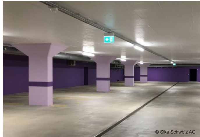
Ceilings and columns freshly restored with FIRETEX Concrete WB.
