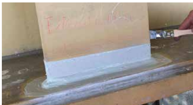
A brush is used to spread the 2-pack coating material evenly.
