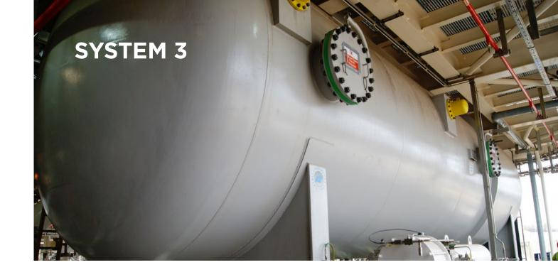
System 3A: Internal lining of tanks for potable water, -20 °C to +40 °C (Carbon steel)
