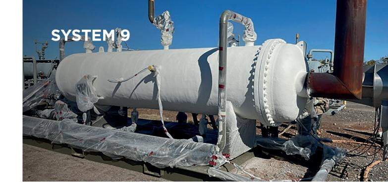
System 9: Offshore and coastal environment, insulated, below -50 °C (Stainless steel, Non-ferrous metals)
