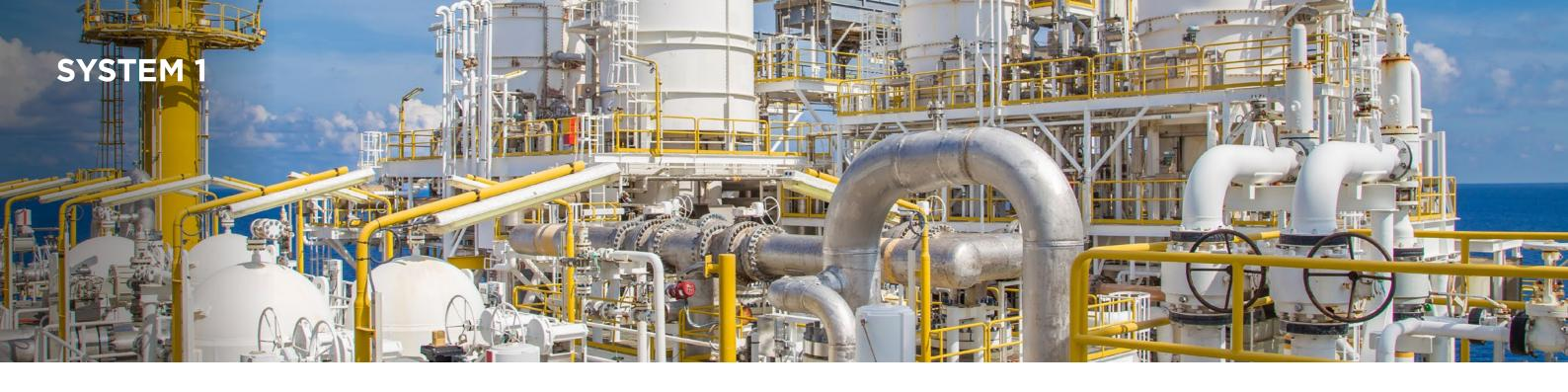
System 1A: Offshore and coastal environment, non-insulated, -50 °C to +80 °C (Carbon steel, with inorganic zinc rich primer)
