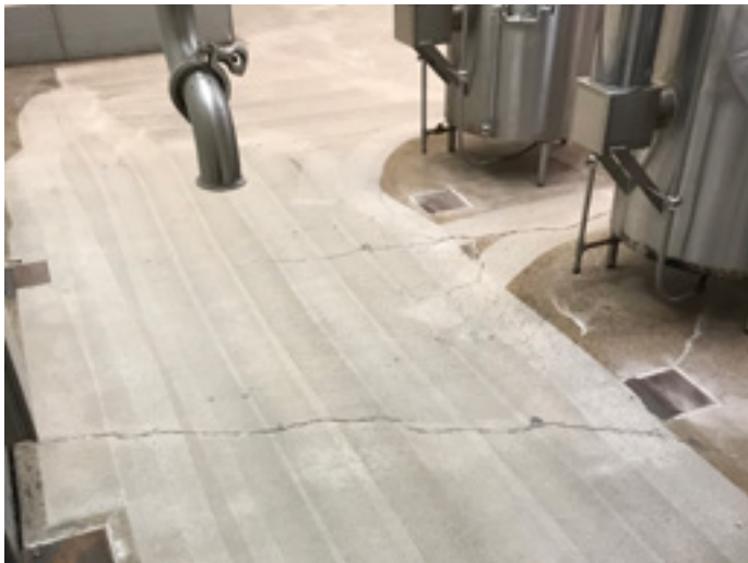
Areas around heavy equipment that vibrates are prone to cracking, particularly at and near attachment points..
