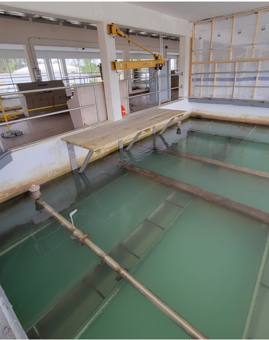
Figure 1. The project centered on rehabilitating six gravity filter basins with varied conditions and coatings, employing advanced methods to extend their life while reducing environmental impact.
