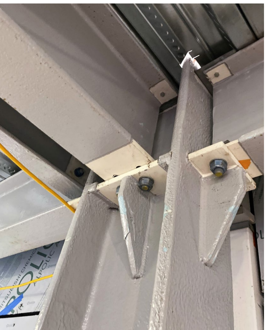
Figure 6. Connection points on structural steel sections featured holdback areas where Puget Sound Coatings applied only a primer in the shop, leaving a flat surface for bolting pieces together. Onsite applicators later applied fireproofing coatings to these areas to ensure protection.
