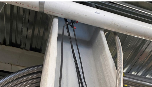
Figure 8. Non-exposed structural steel was coated with just the zinc-rich primer and Firetex FX9502 material, with no topcoat, since the steel would not be visible inside the building.
