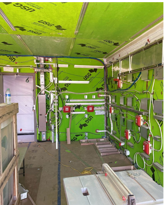
Figure 2. Prefabricated wall and floor panels for 303 Battery arrived onsite with complete heating, electrical and plumbing infrastructure already built in, enabling significant efficiencies in constructing the building.
