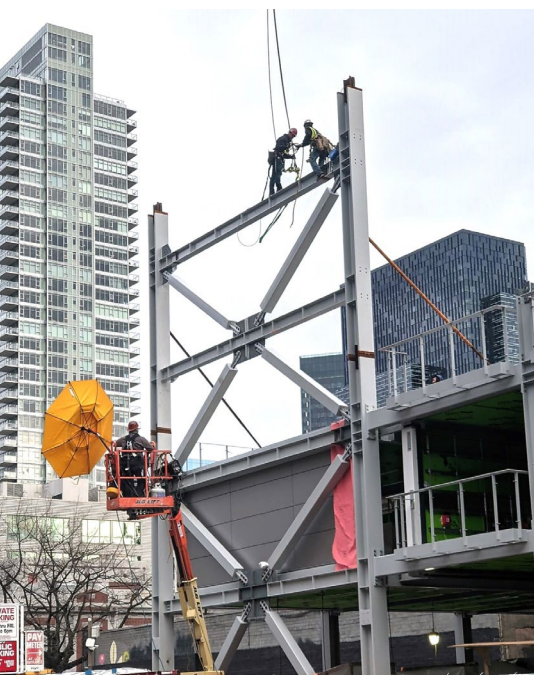
Figure 5. The 303 Battery steel erection team was able to pull fully coated steel pieces directly from delivery trucks and install them rapidly into the structure.
