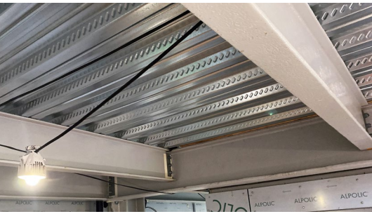
Figure 7. Structural steel that would be visible following construction received a gray topcoat of Sher-Loxane 800 to provide a pleasing aesthetic finish, while any steel that would be covered did not receive a topcoat.
