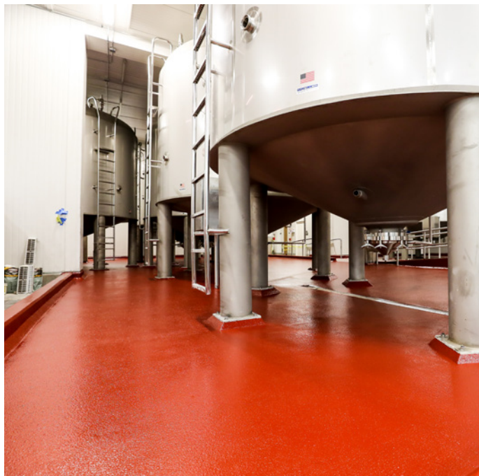
Figure 4. Aggregate broadcast into a resinous floor system provides skid resistance in wet processing areas. An MRO evaluation may flag flooring for skid resistance testing as part of a broader review of facility safety conditions.
