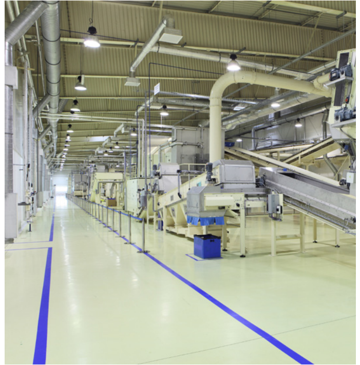
Figure 5. Consistent floor coatings, line markings and color coding are the kind of details a site MRO evaluation can help standardize across a facility — supporting more predictable maintenance and more uniform bid packages.
