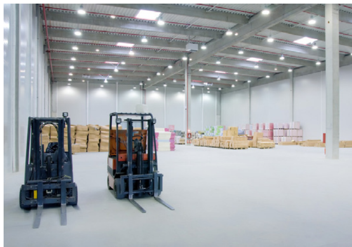
Figure 2. A site MRO evaluation considers the full range of coated assets across a facility — from floors and walls to structural steel and overhead surfaces — and documents how each is performing in actual service conditions.
