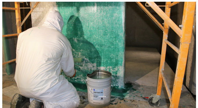
Figure 1 An especially robust protective coating system for MBR basins may include reinforcement with fiberglass matting. In this installation, applicators applied Sherwin-Williams Dura-Plate UHS Clear Laminate as a base layer and then tinted the material green to provide contrast when sealing in a 1.5-ounce fiberglass mat for reinforcement.
