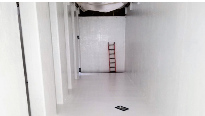
Figure 3 For the final layer of the MBR basin linings, applicators spray-applied Dura-Plate UHS Epoxy White, an ultra-high-solids epoxy amine coating engineered for immersion service that features high-build, edge-retentive properties for superior protection.
