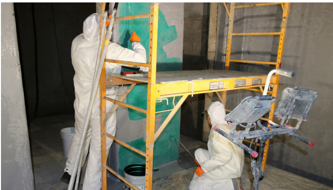
Figure 2 Using aluminum fiberglass rollers, the applicators worked the green-tinted laminate material into the matting to ensure full wetting and proper adhesion.
