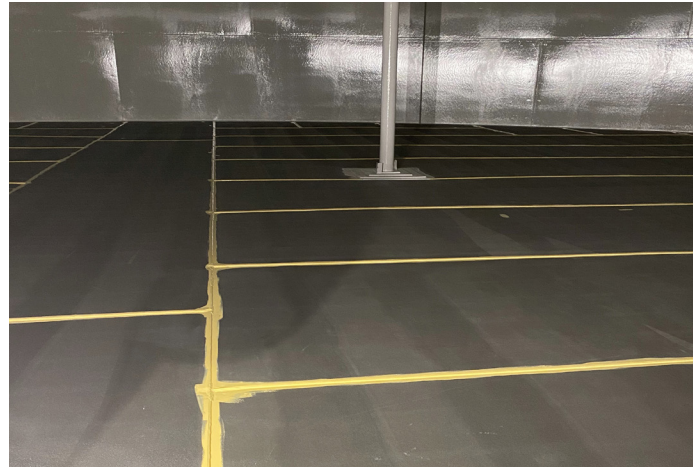
Figure 4 For added protection in steel tanks, applicators commonly apply stripe coats of Dura-Plate UHS Primer, using a combination of brushing and rolling techniques, to ensure full coverage on weld seams, bolts and edges.
