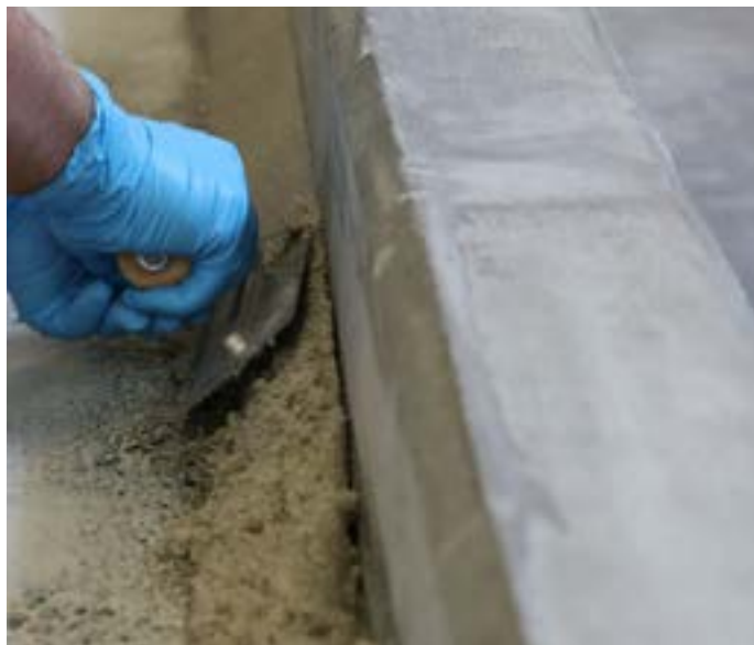
Figure 4. Adding an integral cove base where flooring interfaces with a vertical surface provides a seamless transition that helps direct water and cleaning agents toward floor drains, minimizing standing water and bacteria harborage points.
