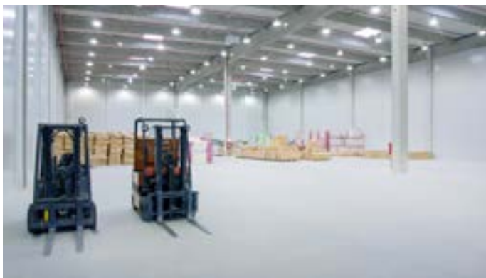
Figure 5. Heavy-duty industrial grade flooring is needed in warehousing, storage and shipping areas to help protect concrete substrates from potential damage inflicted by heavy moving equipment, high traffic, abrasion and impact.
