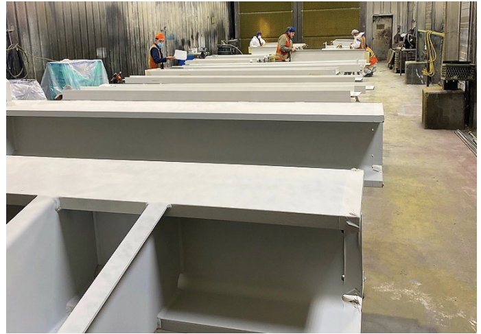
Figure 1. Applying primers and intumescent fire-resistant materials (IFRMs) in a controlled coatings shop environment offers notable efficiencies that can accelerate construction schedules and minimize on-site coatings activities compared to applying all the coatings in the field.
