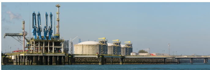
Figure 4. Most full containment tanks made from double-walled carbon steel and insulated with concrete remain uncoated unless the owner prefers a coating for aesthetic purposes.
