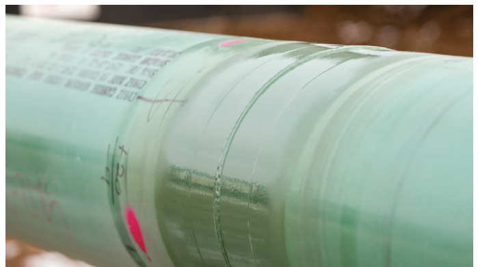
Figure 7. Field-applied, powdered fusion-bonded epoxy (FBE) coatings provide excellent integrity with shop-applied mainline FBE coatings for outstanding resistance to impact damage, abrasion, chemical immersion and cathodic disbondment.
