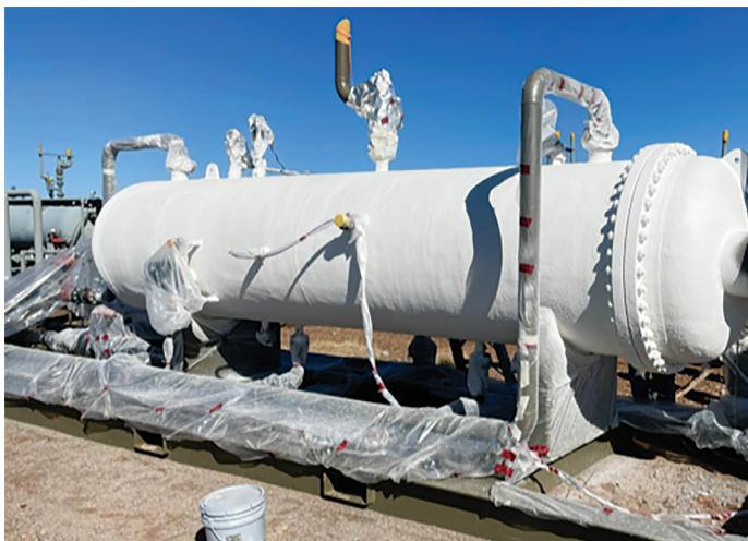
Figure 3. Using a thermal insulative coating system with an advanced energy barrier to curb the transfer of heat on process vessels and other assets can help LNG producers forgo the use of traditional cladded insulation systems while eliminating CUI altogether.
