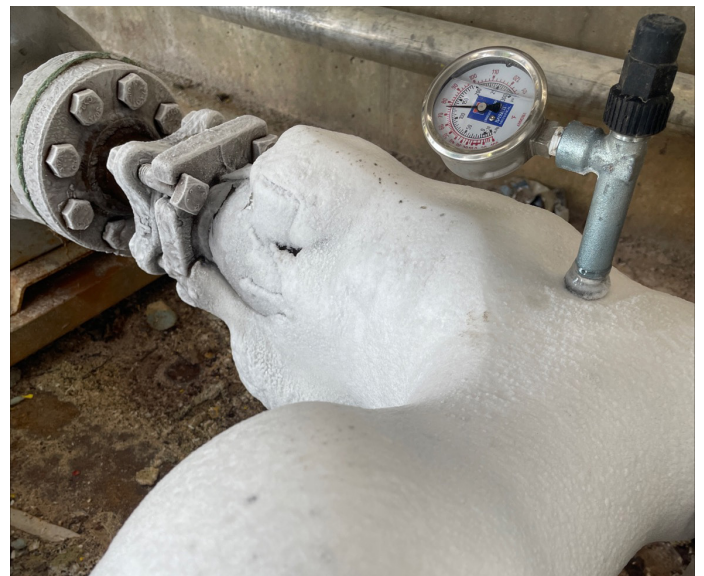
Figure 5. Condensation and ice can form on the exterior of assets experiencing significant temperature differentials between their interior contents and the ambient air.
