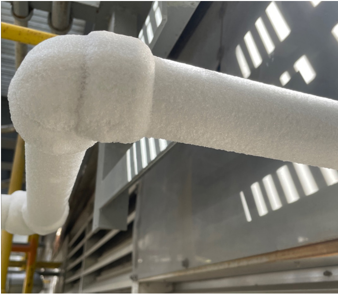
Figure 3. Using a thermal insulative coating on various assets such as process piping allows pipeline operators to remove physical insulation systems, while maintaining process heat, minimizing condensation and eliminating CUI in the process.
