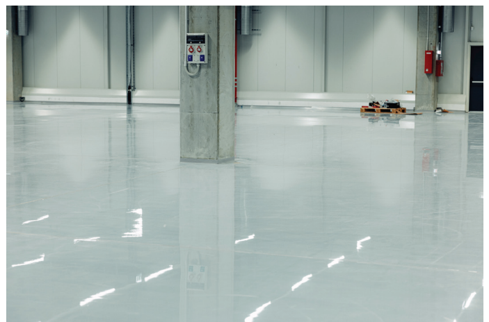
Figure 3. Flooring throughout a semiconductor fabrication facility needs to be highly durable and rated for the traffic and chemical exposures it will encounter.
