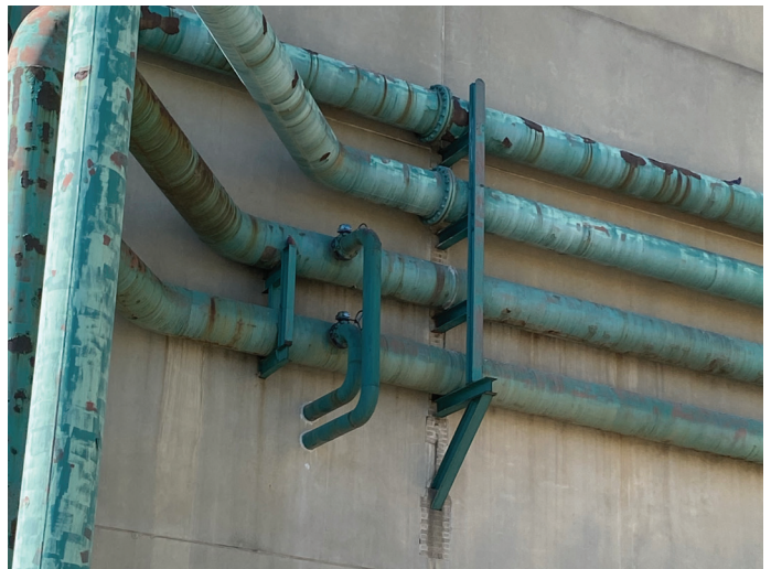
Common in many plant environments, long stretches of insulated process piping are notorious for experiencing CUI. Water nearly inevitably breaches their insulation systems, leading to diminished insulating capacity and exacerbated CUI.
