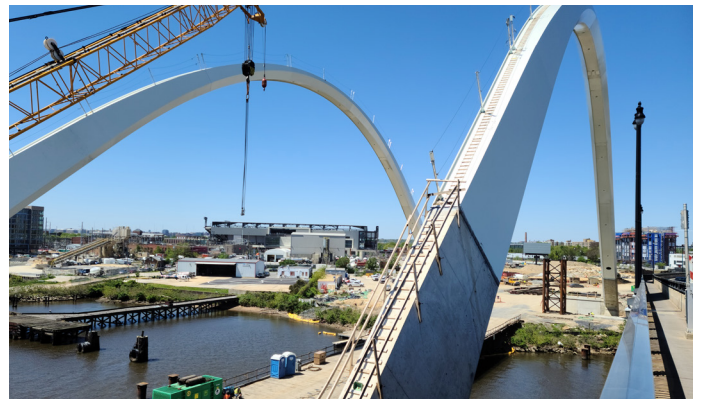
Figure 2. Structural steel for the Frederick Douglass Memorial Bridge in Washington, D.C. was shop coated and finished with a polysiloxane topcoat for long-term color and gloss retention. Image courtesy of Champion Painting Specialty Corp
