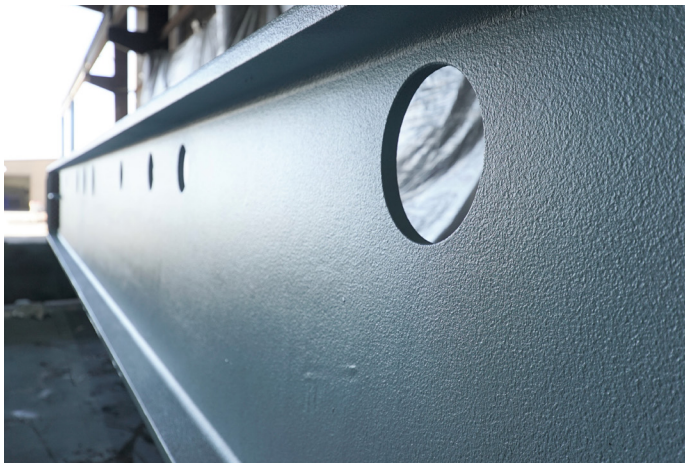
Figure 5. Intumescent fire-resistive materials (IFRMs) comply with outgassing, low dusting and environmental tolerance requirements that are essential for food and beverage cleanroom environments.
