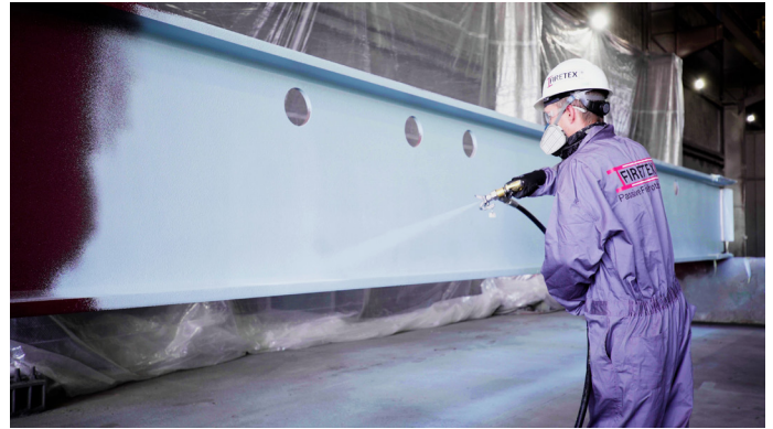
Figure 6. Off-site application of epoxy intumescent fireproofing before constructing a food and beverage cleanroom environment eliminates potential numerous on-site challenges.
