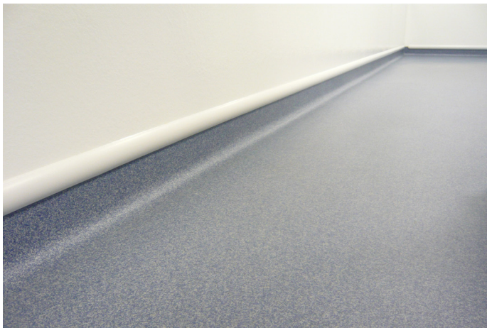
Figure 1. Cove bases provide a seamless transition between floors and wall surfaces, ensuring ease of cleaning by eliminating gaps or crevices where dirt, debris or microbial contaminants could accumulate.
