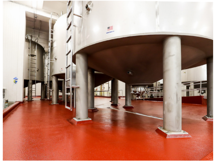
Figure 2. An auditor may suggest incorporating skid resistance into flooring to reduce the potential for slips and falls and enhance worker safety.
