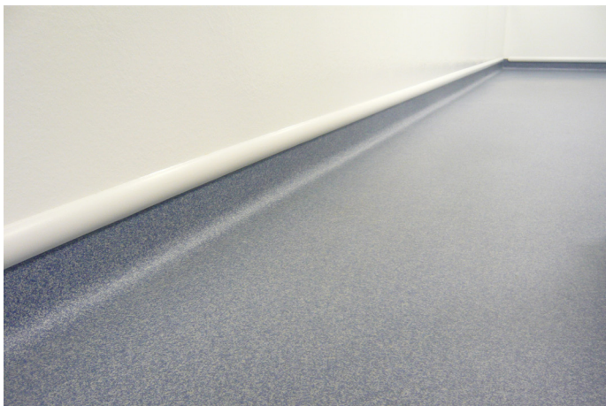
Figure 1. Cove bases create a seamless transition between floors and wall surfaces to enable ease of cleaning, as no gaps or crevices will exist where dirt, debris or microbial contaminants could accumulate.
