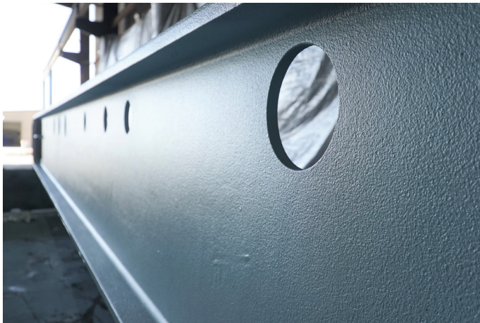
Figure 5. Intumescent fire-resistant materials (IFRMs) meet requirements for outgassing, low dusting and environmental tolerances in cleanroom environments.
