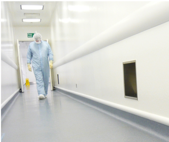
Figure 4. Wall systems in sterile environments like cleanrooms need to be highly cleanable to minimize contamination potential, as well as durable to withstand the rigors of harsh cleaning protocols and prevent damage from impacts and abrasions.
