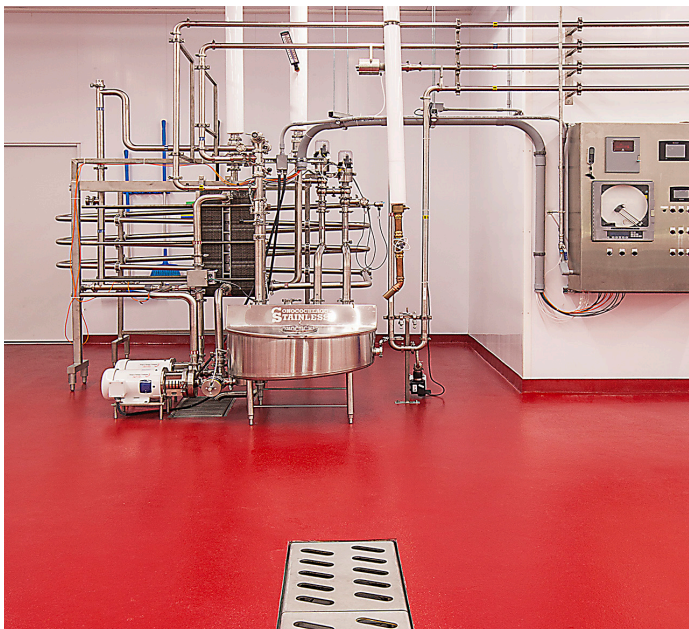
Figure 3. In areas subjected to frequent washdowns, moisture tolerant, chemical and thermal shock resistant coating systems can be used to correct the floor slope for proper drainage. This helps avoid unhygienic puddling and improves safety, as well as cleaning efficiency.
