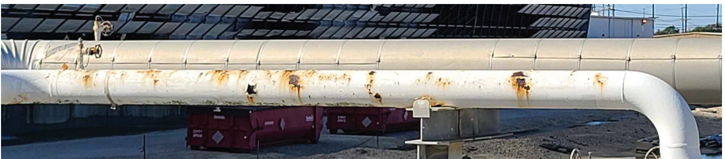
Figure 1. Fallout from chemical plant operations settles onto steel assets, and mixes with water to accelerate coating degradation and promote undercutting corrosion.
