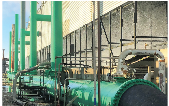
Figure 3. The new MIO-enriched coating system for fallout areas promotes durability from the top down, with a Sher-Loxane 800 topcoat, Macropoxy 267 intermediate coat and Corothane I MIO Zinc Primer.
