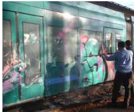
DURING: Due to the size of the project the GRS solution was spray applied for easy application.
